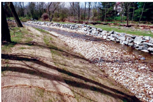
Figure 3: Restored section of MNBK in Cromwell Valley Park in the foreground, with the original stream channel visible in the background (Source: Doheny et al., 2012).
