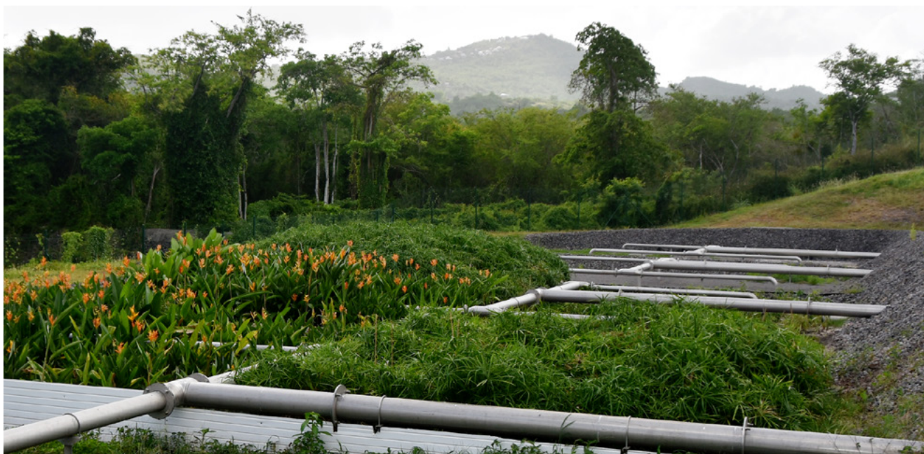
Figure 1: Taupinière unsaturated/saturated French VFTWs planted with Heliconia psittacorum and Cyperus alternifolius
